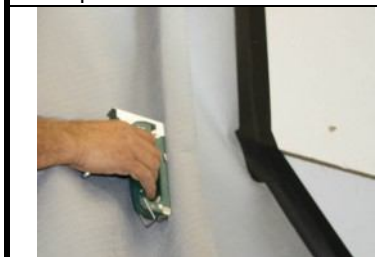
12.10 fix the membrane on valley counter batten with the staples
