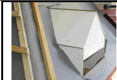
12.1 small dormer on the roof
