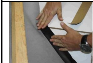
12.4 stick the membrane overlap on the side of the dormer
