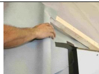
12.9 apply membrane over the valley counter batten
