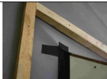
12.8 detail of sticking – ridge of the dormer
