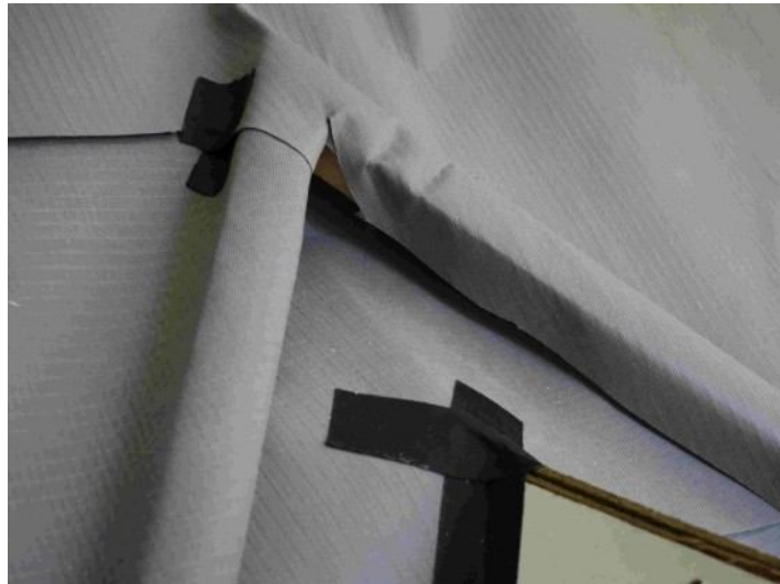
Detail of membrane overlaps sticking at dormer's ridge and membrane fixing over valley counter battens
