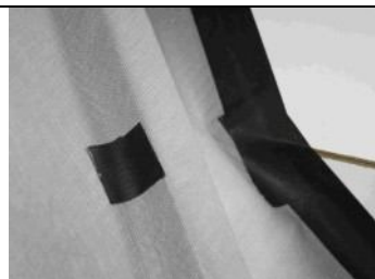
12.11 stick the tape JTD SP SUPER over the staples
