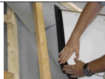
12.6 stick the membrane overlap on the roof of the dormer
